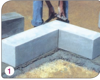
1 Conventional mortar used for laying first course of blocks
