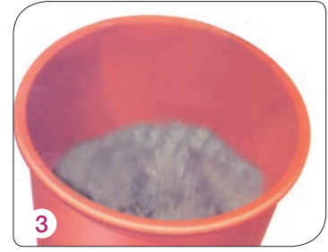
3 Allow the resultant wet mortar to stand for 5 mins for the additives to dissolve. Use the mix within 20-30 mins for best results
