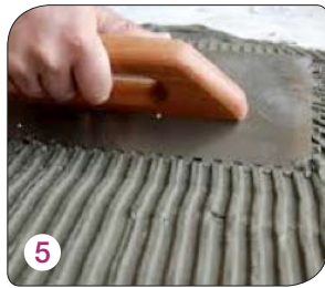
5 Ensuring 3 mm layer and complete filling of joints
