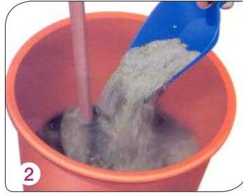
2 In 10 -12 l of water, add 40 kgs of Aerocon Smartfix Jointing Mortar. Stir mix continuously for 5-10 mins by using electric mixer or by hand to obtain homogeneous lump-free mix
